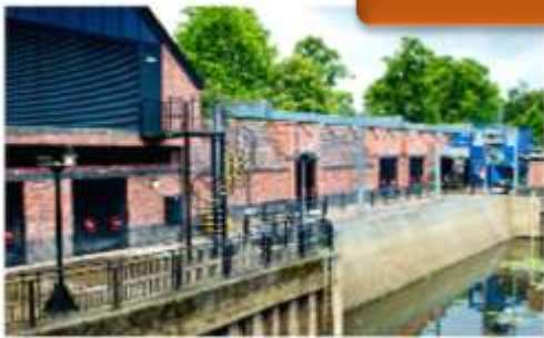
A flood defence wall
