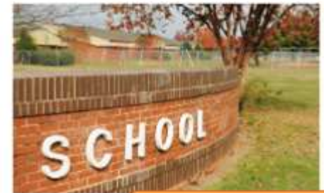
A wall surrounding a school
